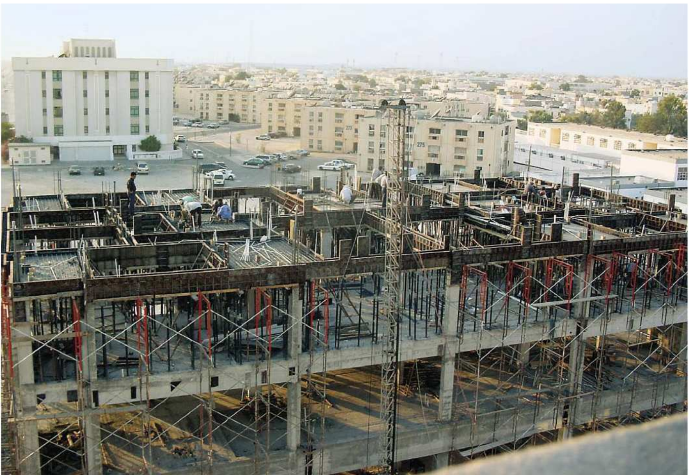
Wohnanlage, BRN-Bahrain; Fa. Tower Marketing & Contracting W.L.L., BRN-Bahrain
