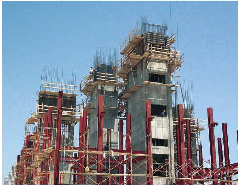
18-stöckiger Hotelkomplex in Seef, BRN-Bahrain; Fa. Dadabhai Construction, BRN-Bahrain
